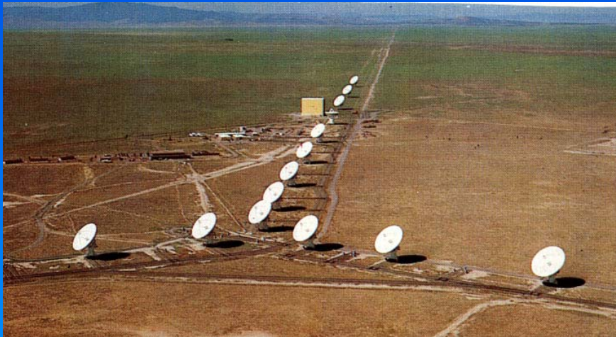
The VLA (Very Large Array), a set of 26 dishes, each of 25 m, which can be moved along rails stretching 15 miles from the centre
