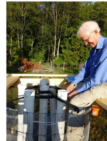
Attaching the PVC pipes to metal frame mounted on top of bioreactor cage. The pipes are pulled out 24 hr after loading, leaving behind 6 air channels to provide oxygen to the rapidly reproducing bacteria.
